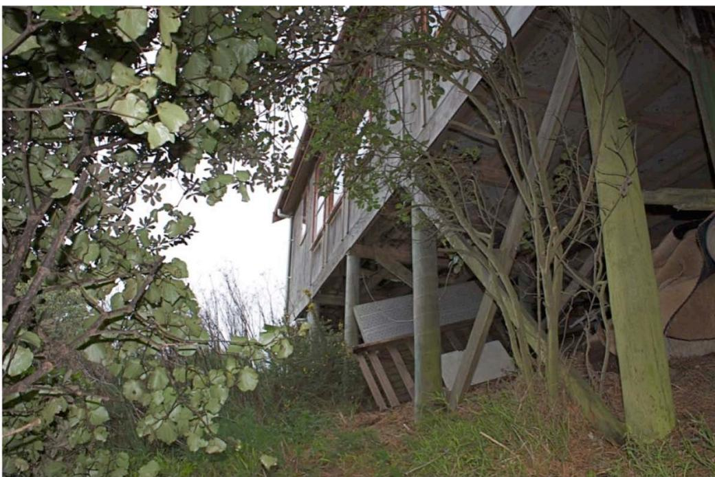
Figure 6: timber supports for the building structure
